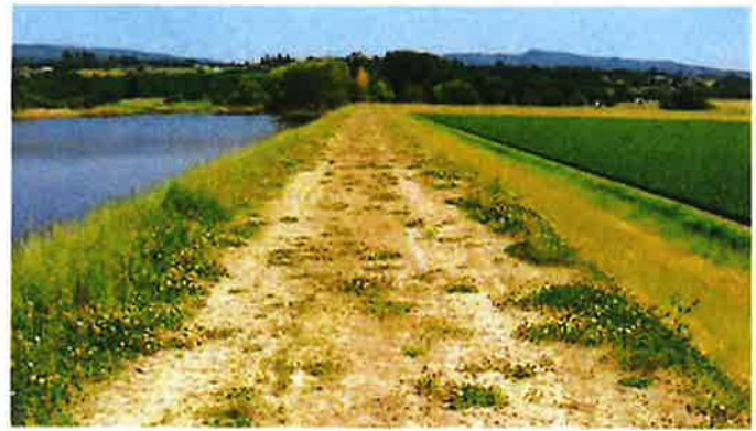
A levee protects adjacent farmland from flooding
